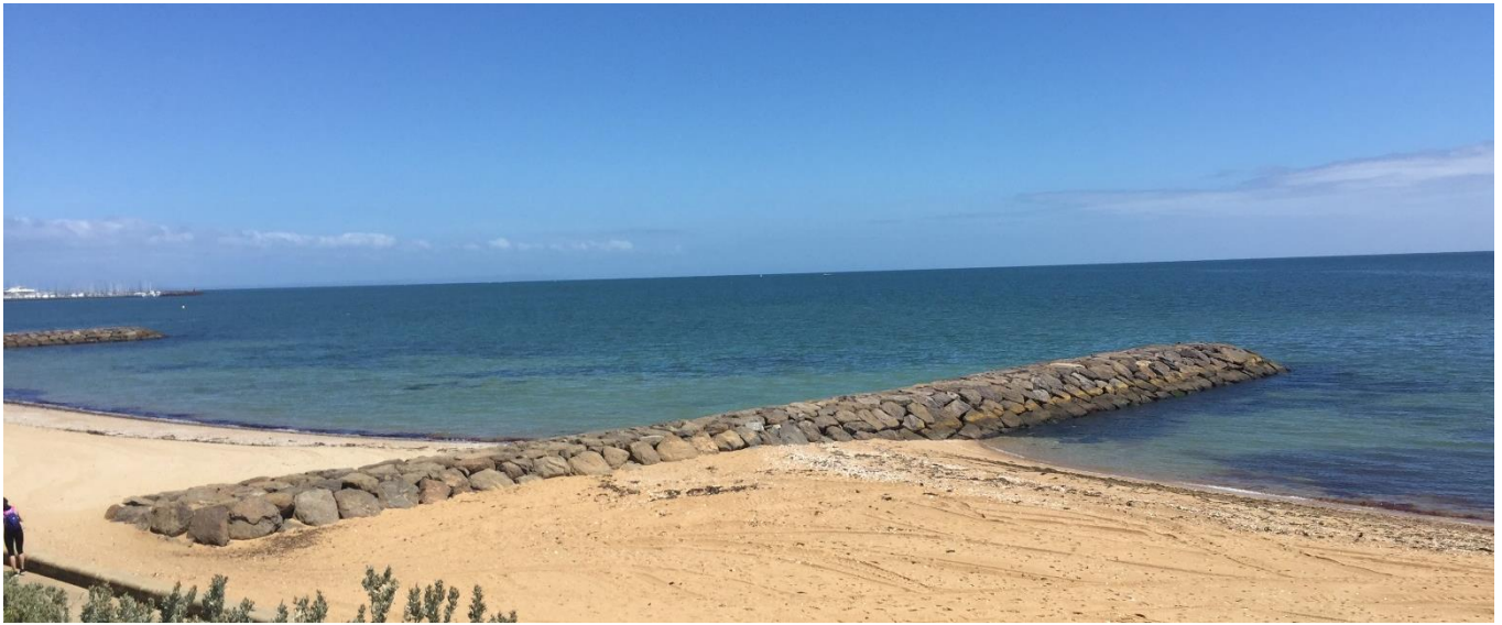
Figure 5: Small groyne (80m long) installed at Brighton beach.
