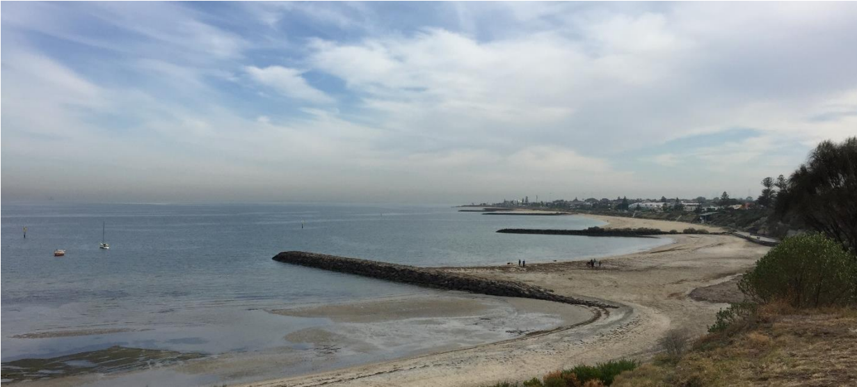
Figure 2: Large groyne installed at Hampton Beach with a large-scale renourishment. This groyne is 143m long, with approximately 50m partially buried. Groynes at Mount Martha would need to be 1.5–2 times longer.
