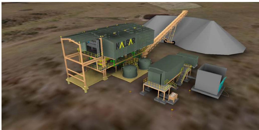
Figure 7 Centrifuge building and cake stockpile
