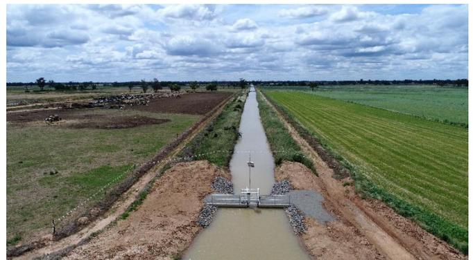
**Figure 1: The Connections Project has modernised irrigation delivery infrastructure to reduce water losses, with works completed in all six irrigation areas of the GMID.**
