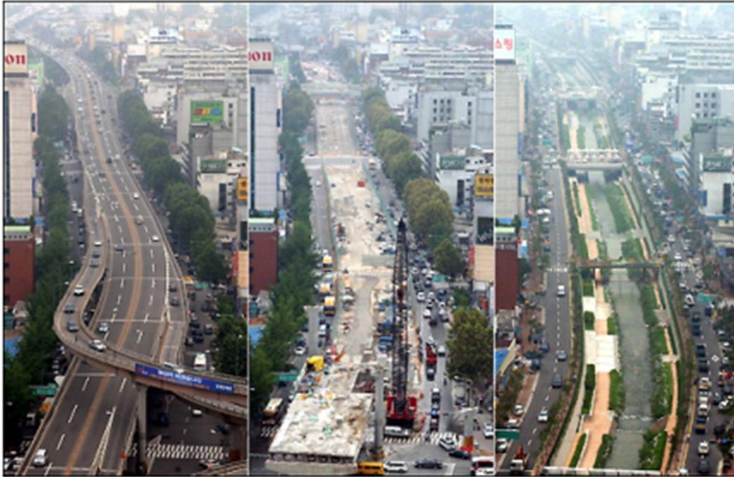
Photos showing the freeway, its destruction, and the resultant new setting. Image source:
