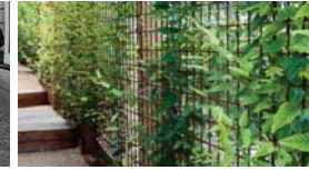
Timber and steel reinforcing wire as a trellis for climbing plants.
