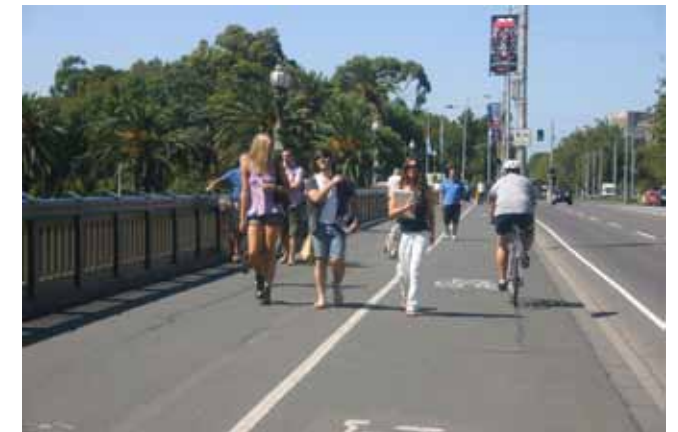
Figure 12 – Linemarking and pavement symbols are not considered sufficient to separate cyclists from pedestrians.
