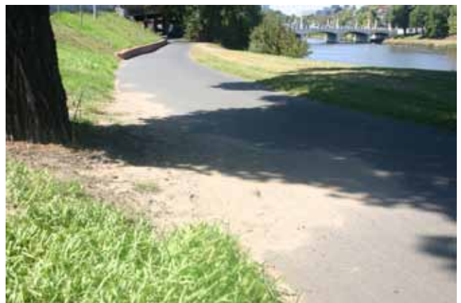
Figure 15 – Deep sand such as this can be hazardous to cyclists, especially in shaded areas.
