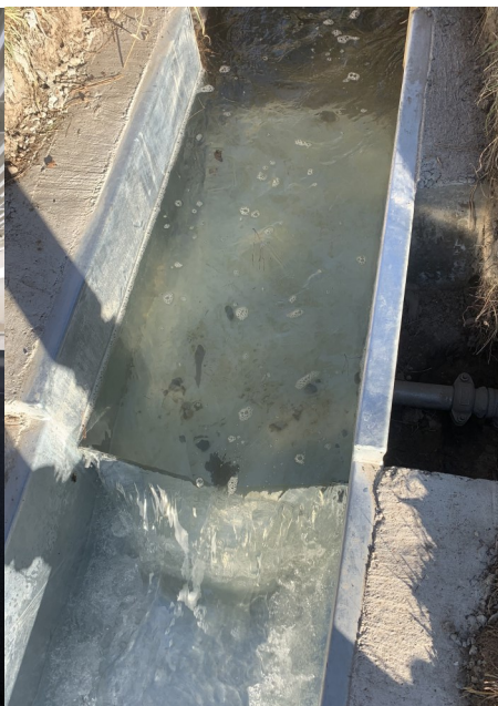
The new weir under construction.
