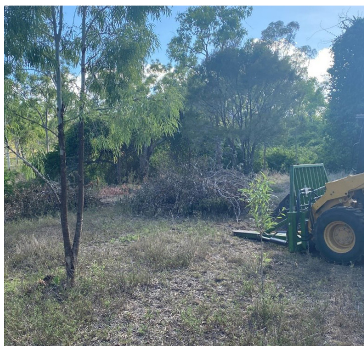
Rubbervine along a creek line cleared using an Auscrimper sucker puller.
