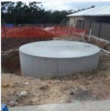
SOUTH SOLITARY DISPLAY HOME UNDER CONSTRUCTION, WITH OUR 20,000 LITRE TANK UNDERNEATH THE GARAGE FLOOR
