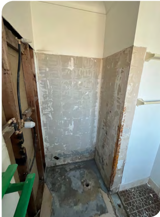
1. Removal of wall tiles and floor
