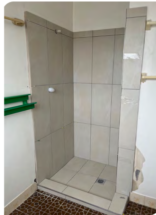
3. Retile walls and floor
