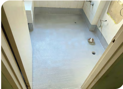
1. Remove and waterproof the bathroom floor and first row of tiles
