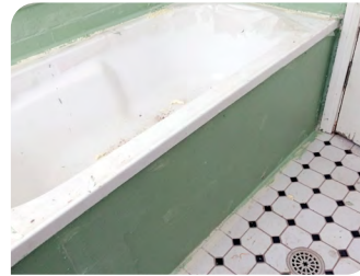
3. Bath installed and waterproof applied over bath lip
