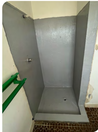
2. Walls & floor waterproofed
