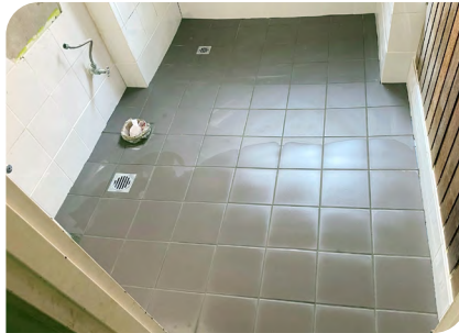
2. Bathroom floor and bottom row is tiled and grouted.
