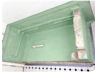
2. Waterproof the bath area
