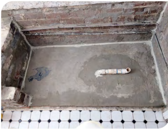
1. Bath removed and prepared for waterproofing
