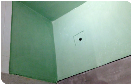
3. New shower area waterproofed
