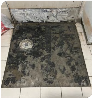
1. Demolish bottom row and floor; primer and backing rods
