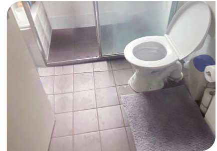
3. All PC items installed, and junctions sealed with a flexible anti-mould sealant.
