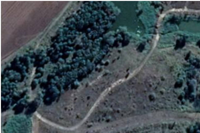
Photo 25. Two adjoining farm road crossings of the lower reaches of the system downstream of the Bruce Highway utilise piped culverts. These generate high flow velocities that would act as fish passage barriers under a broad range of flow conditions.
