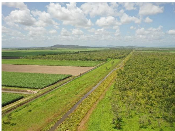
Photo 53. Sunwater drain (RB1) within the BHWSS (Reach 1, Figure 9). These drains form the upper catchment of the Collinson's Lagoon system. They are essentially a long linear wetland. Their existing ecological values and function is limited. Grass weed rafts exported from these drains in high flows create downstream flood risks.
