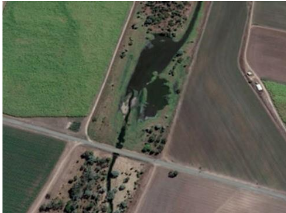
Photo 45. This smaller lagoon downstream of Rose Road on the main drainage line (Reach 6, Figure 9) represents a sediment depositional zone. Colonisation of sediment beds by aquatic grasses serves to further occlude flows (M11).
