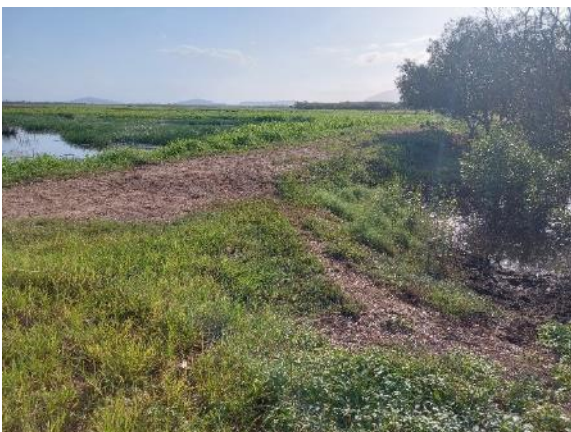
Photo 6. Earth bunds provide tidal exclusion and increased freshwater pasture pondage on the downstream margins of the Corrick Plains Nature Refuge. These bunds separate tidal mangrove from freshwater pasture.
