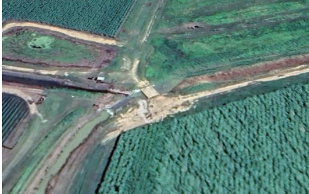
Photo 1. Sunwater drain RH5 conveying catchment runoff from the BHWSS over a small in-channel weir into a drain leading to the upper Horseshoe Lagoon system (right).
