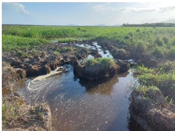
Photo 7. Where high flows damaged bund walls the aerial extent of post wet season-ponded freshwater wetland could be reduced. Rock armouring of these areas using a rock ramp fishway configuration could both reduce erosion and provide fish passage.
