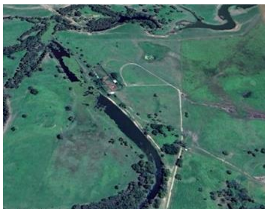
Photo 14. Clearwater distributary lagoons isolated from aseasonal tailwater inflows.
