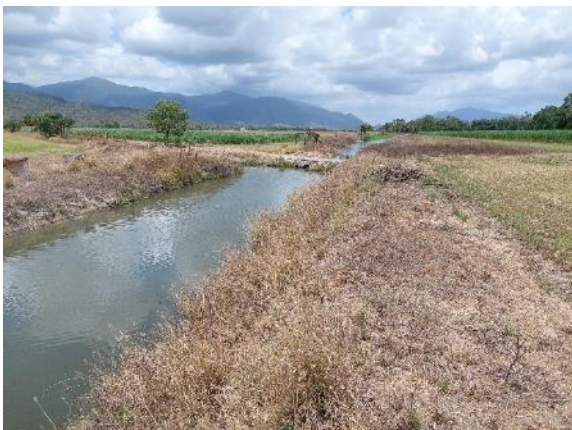
Photo 3. Irrigation recycle pit within a large capacity channel that forms part of a farm drainage system in the upper catchment of Ironbark Creek. Promoting revegetation of farm drain and increased detention of runoff would help to improve water quality and reduce soil erosion risks.
