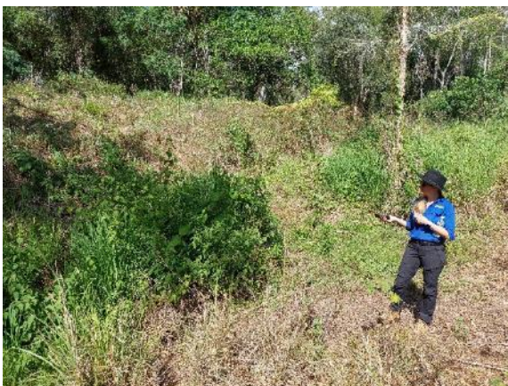
Photo 1. Power line access track across the distributary channel break out from the Houghton River to Ironbark Creek has raised the channel invert level and the flow height required to initiate channel flow.
