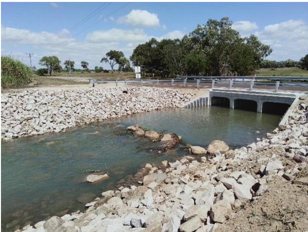
Photo 13. Rock ramp fishway installed below culvert on Five Ways Road reducing culvert flow velocity.
