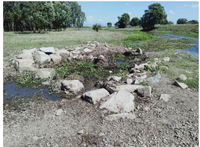
Photo 12. Rock ramp fish bypass established adjacent to a Lower Burdekin Water control structure.
