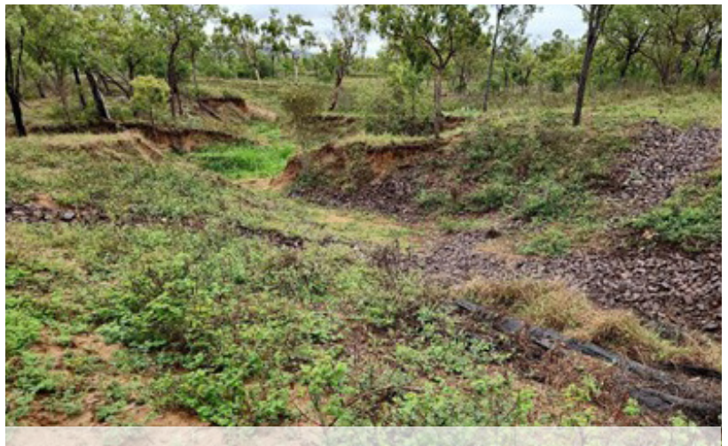
October 2022 In the lower sections of the main gully channel, walls were stabilised, and rock structures were installed to slow water flow and reduce erosion. This method provided an effective solution while minimising costs by avoiding the need for extensive reshaping of the entire system.
