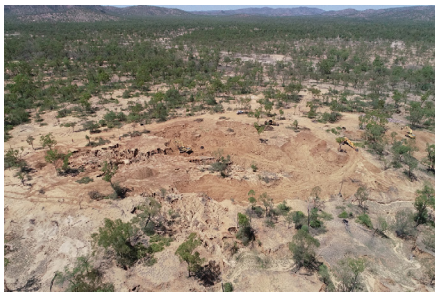
Aerial view of the site during remediation.
