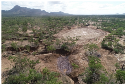
Aerial view of the site right after remediation was completed.
