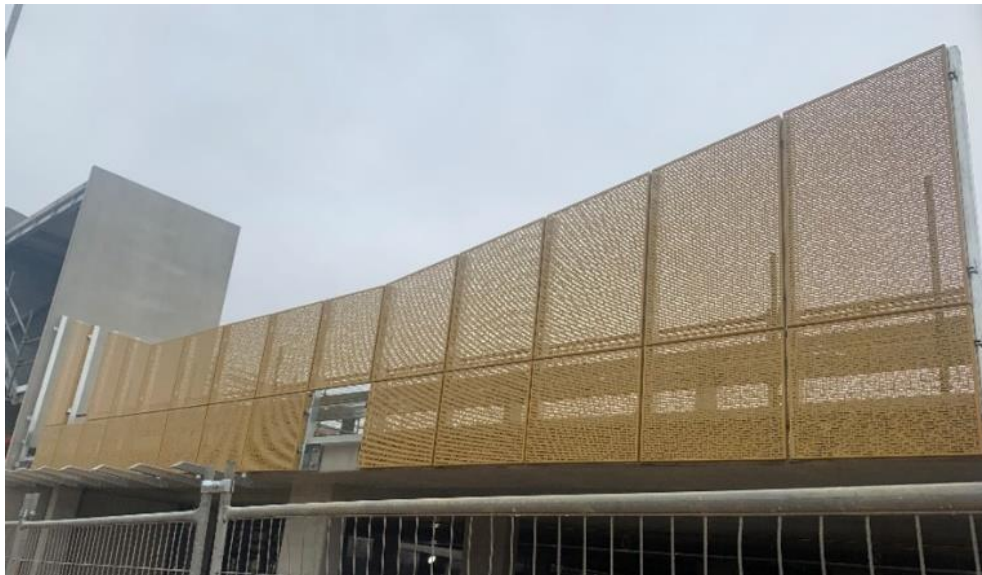
Façade works commenced in November 2021
