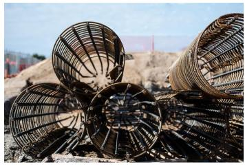
The steel reinforced cage that is placed into the pile
