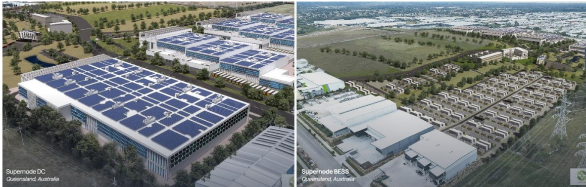
Supernode Data Centre and Battery at Brendale ( https://supernode.com.au/ )
