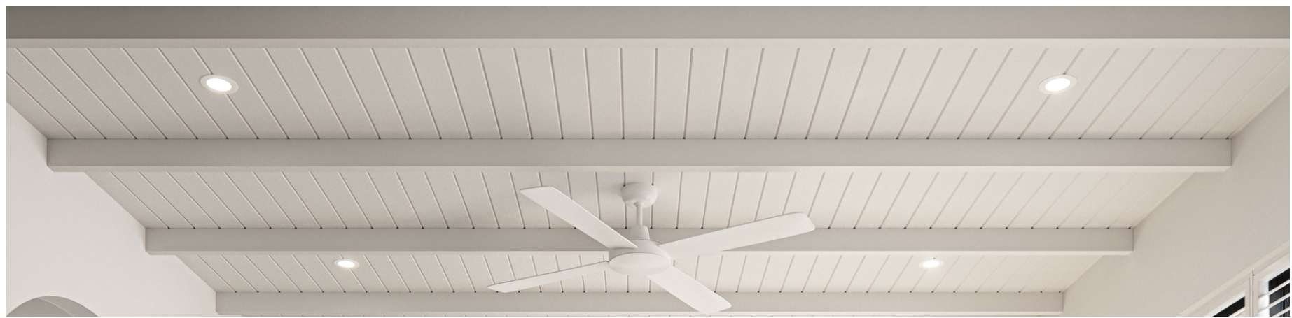
CEILING FEATURE VJ CLADDING WITH BATTENS
