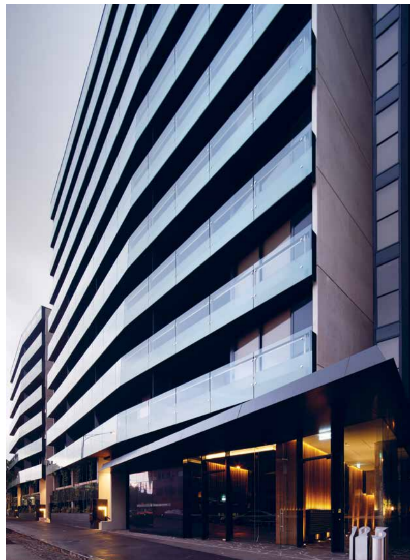
Bravo Apartments CARLTON, MELBOURNE
