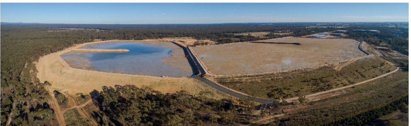
Figure 4. Aerial image of FGM's TSF1 and TSF4 facilities
