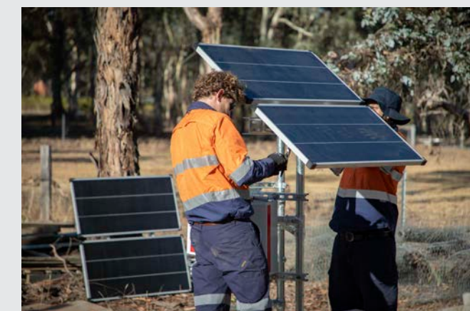
Institute of Mine Seismology (IMS) installing new surface ground vibration monitors as part of a network expansion.
