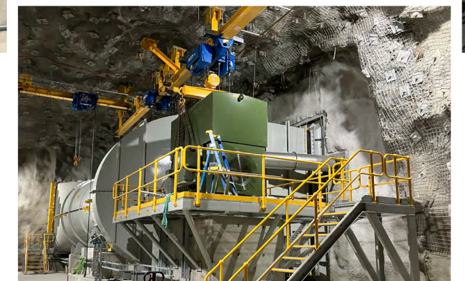
Above: The newly installed underground ventilation fan in chamber 1 and chamber 2 (inset).
