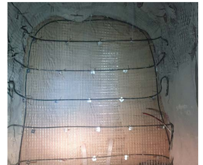
Step 2: Cloth and steel mesh installed.
