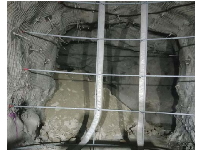
Step 1: Steel frame is installed.
